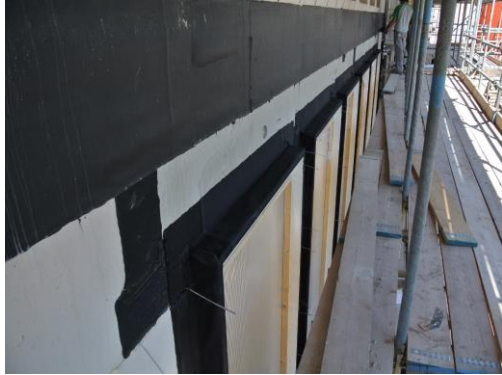
▲ sealing the window perimeter
