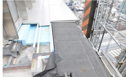
▲ sealing the vertical-to-horizontal transition location
