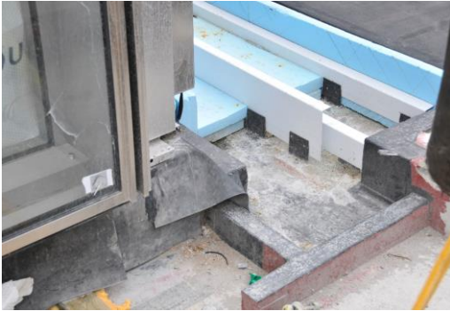
▲ sealing the window perimeter, window/starter sill
