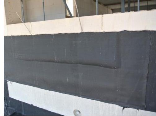
▲ sealing the joint between floors
